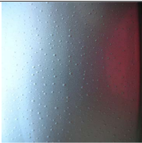
Figure 7. Example of blistering on finished surface
