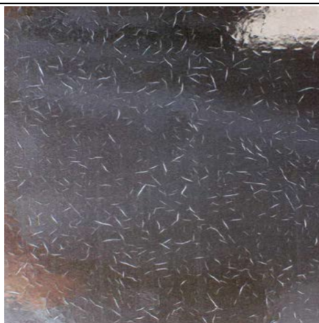
Figure 10. Example of checking on a finished surface
