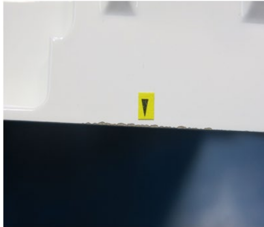
Figure 4-24 – Tape line chipping
