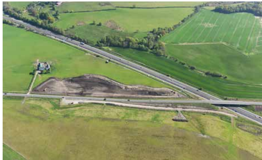
Work continues to progress at M8 junction site
