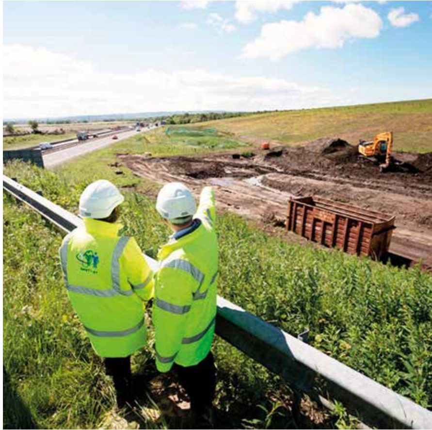
Overseeing the development of the new junction
