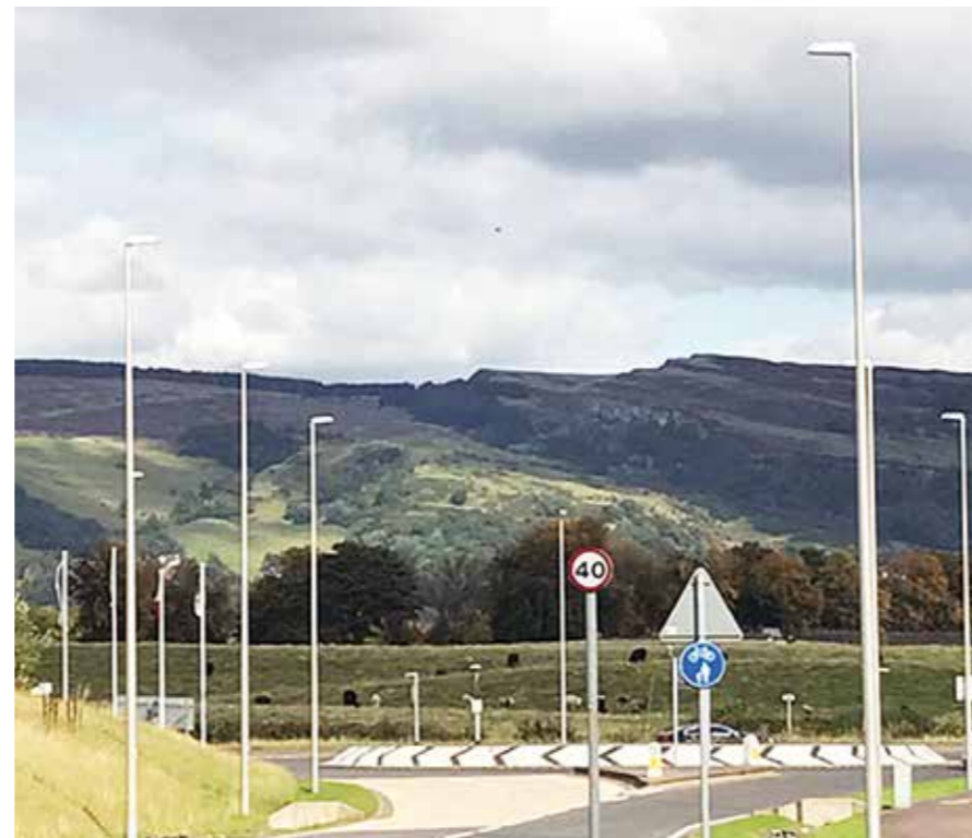
The new LED street lights at the top of Slateford Road
